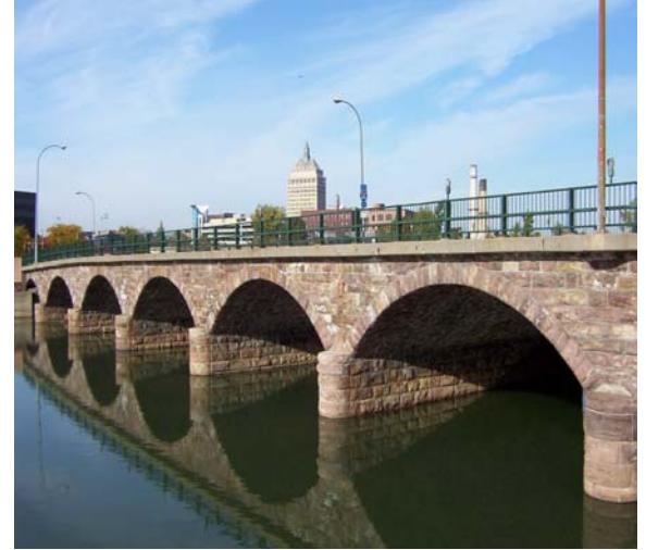
The Andrews Street Bridge
