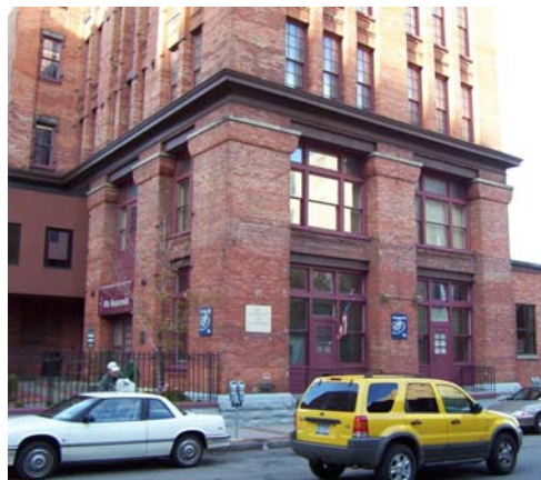
The Ellis Building
