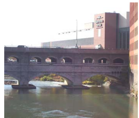
Broad Street Bridge
