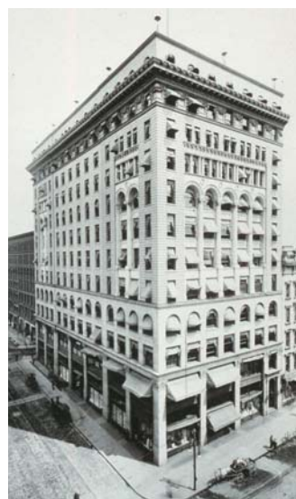
Granite Building circa 1898
