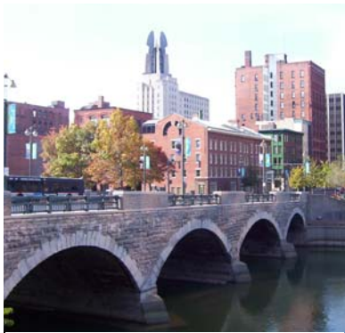
Main Street Bridge.
